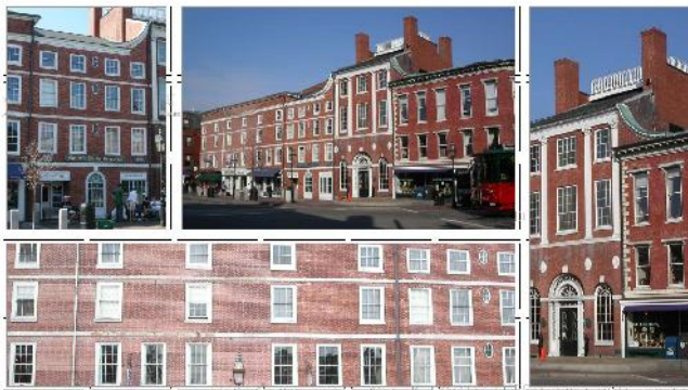
645 CONGRESS STREET | FACADE TREATMENT STUDIES | Four Market Street | May 15, 2004 Portsmouth, New Hampshire 03801 | 603-480-0274 Fax: 603-480-0247 | McHenry Architecture | Scale: 1" = 30'
